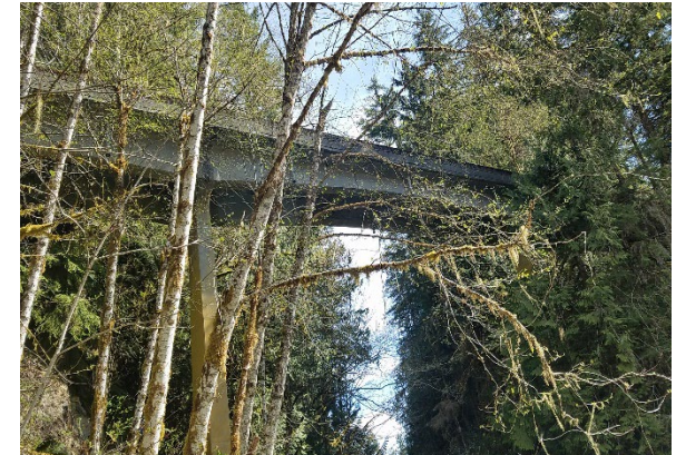
Looking Under the Finney Creek Bridge
